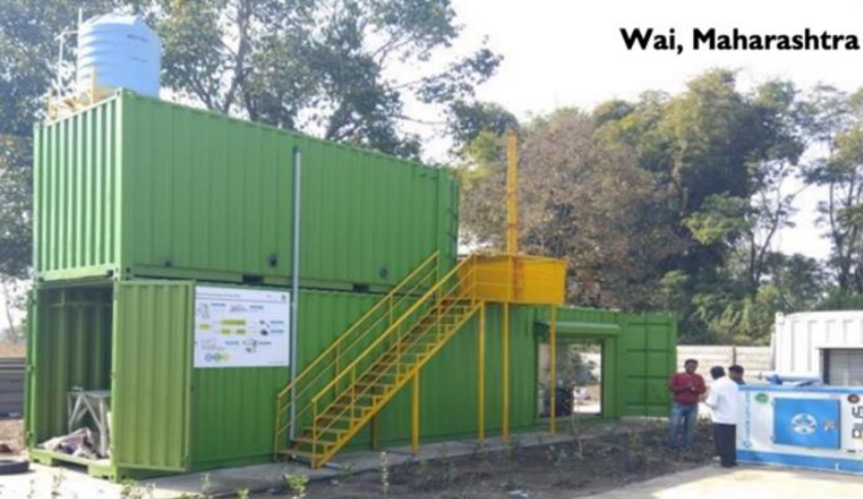
Figure 3.2-3: Faecal Sludge Treatment Plant (FSTP) in the city of Wai (Source: CWAS, CEPT University)
