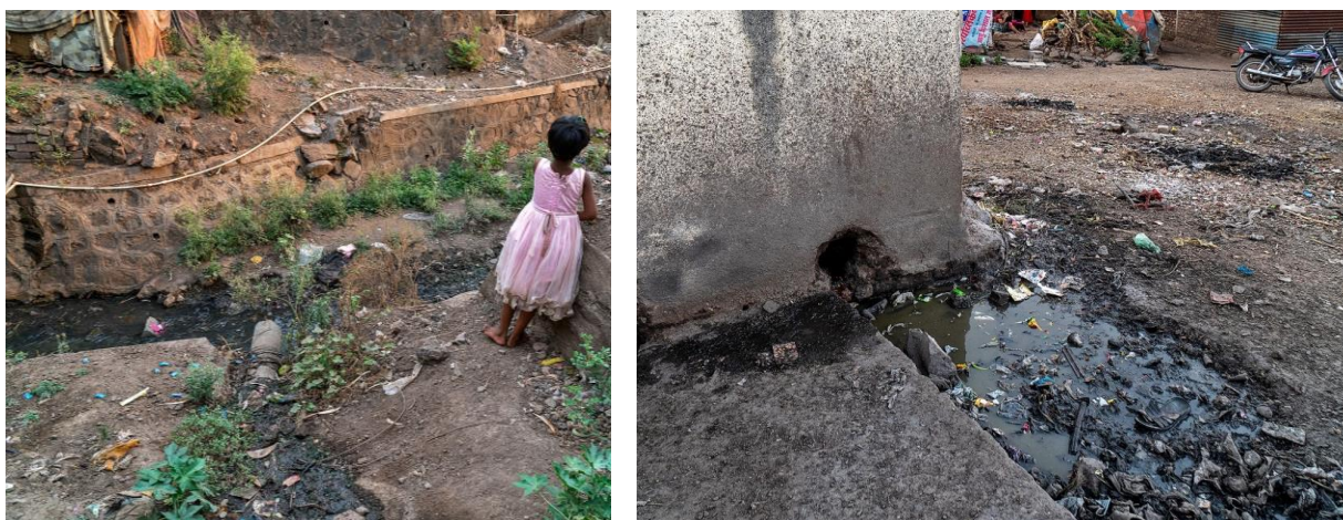
Figure 6.2-2: Open Surface drains in Wai
